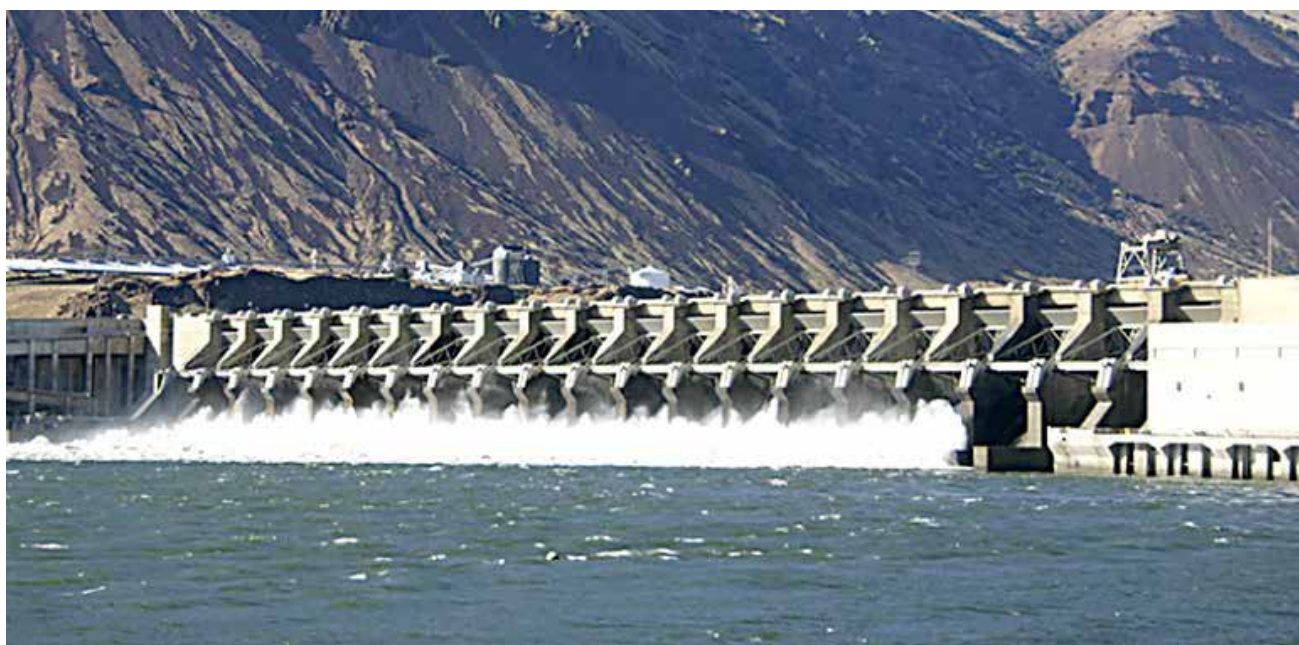
Figure 2. Gaj hydroelectric power plant
