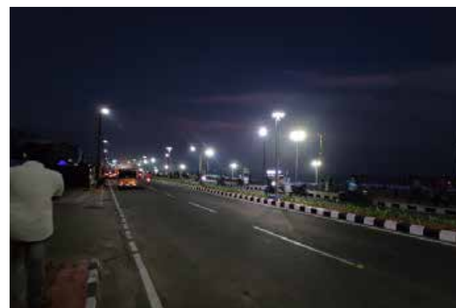
Plate 14. Self lighting and self dimming solar powered street lights at Visakhapatnam
