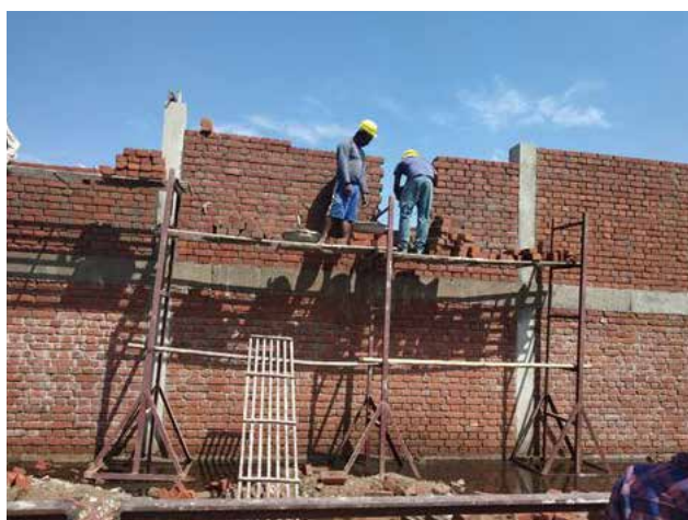
Figure 10 - Image showing the construction of the compound wall (Source: CSCL)
