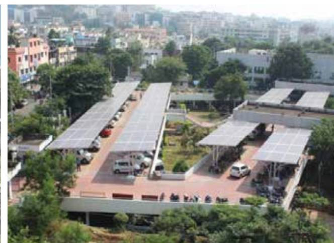
Plate 11. Solar Panels in Parking at GVMC headquarters
