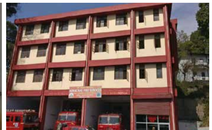
Figure-9: Fire station with trees on both sides creating shadows Source: Rooftop Solar detailed project report
