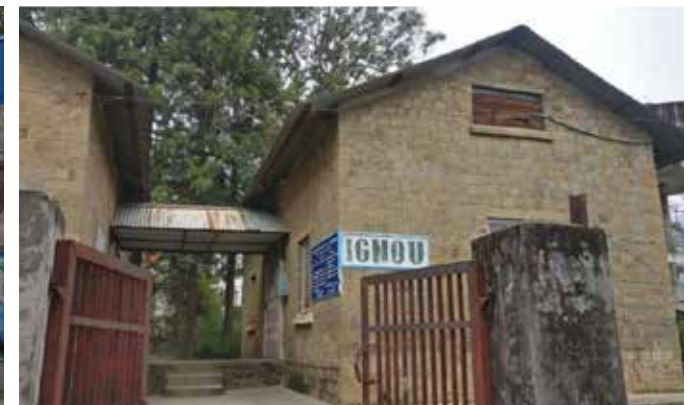
Figure-12: IGNOU building with small roof area and inappropriate orientation Source: Rooftop Solar detailed project report
